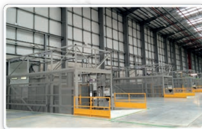
OUR DOUBLE DECK LIFTS CAN ALSO BE FITTED INTERNALLY, IN PRE-CAST SLOTS IN THE WAREHOUSE FLOOR, WITHIN 1-2 DAYS
