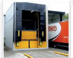
Wheel Guides Aligns vehicles on dock
