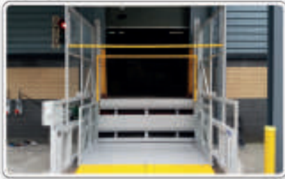
DOCK LIFT BETWEEN RAISED DOCKS AND YARD
