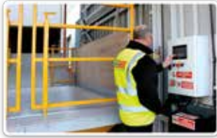
HMI TOUCHSCREEN CONTROLS – WITH RAPID-DIAGNOSTICS* PICTOGRAM AND LIVE PLANT STATUS OVERVIEW
