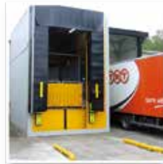
▲ Wheel Guides Aligns vehicles on dock
