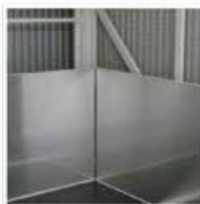
Aluminium Lining 2mm lining beneath handrails
