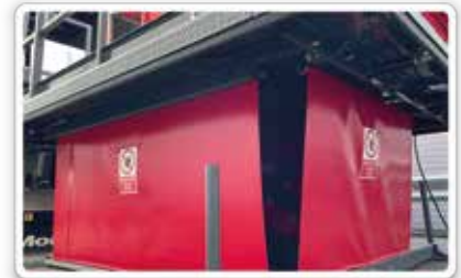
▲ Safety Curtain Prevents access under platform when lift is raised
